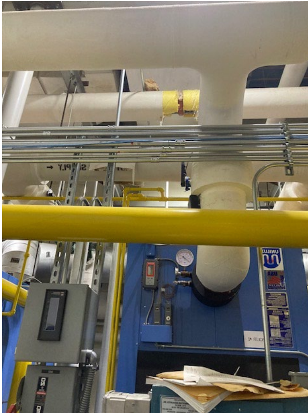
Leaking 6" connection (Rev 2 added pictures)
